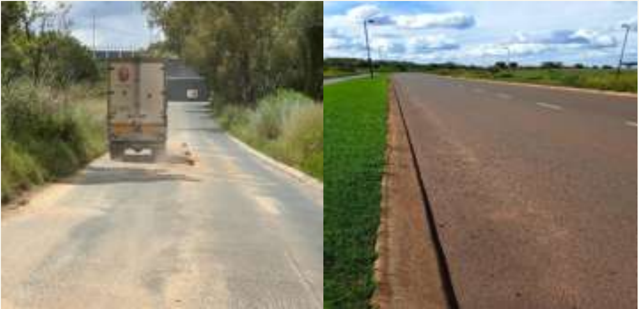
Road built using polyroad technology
