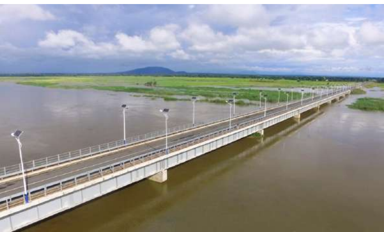
Magufuli Bridge at the Kilombero River in Morogoro Region. The bridge is 384 metres long
