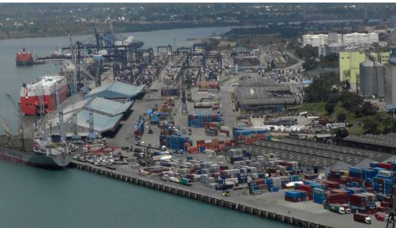
A birds eye view of the Port of Dar es Salaam whose expansion has already been completed, enabling large ships to dock at the port.
