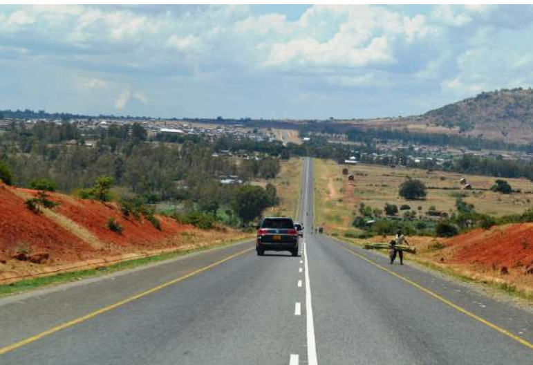
Vehicles seen cruising the 112 km Sumbawanga-Matai-Kasanga Port road in Rukwa Region whose construction to tarmac level has been completed.
